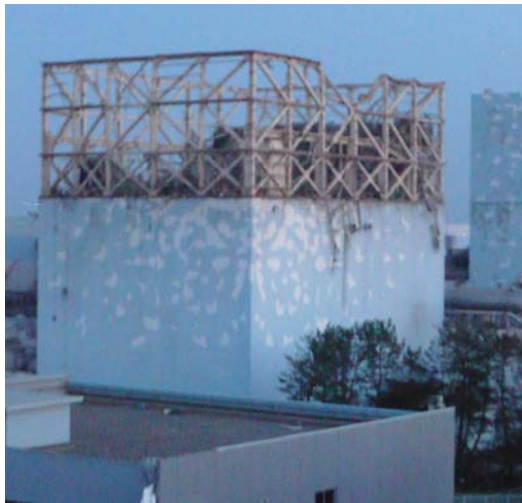
Figure II-2-26 Condition of Reactor Buildings, Units 1 to 4, Fukushima Dai-ichi NPS
