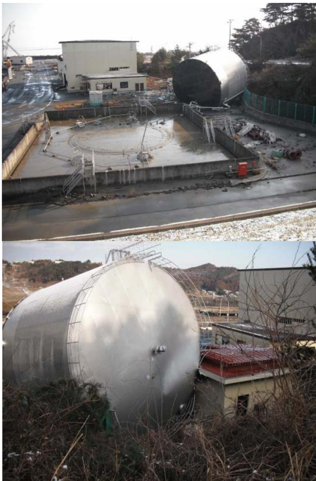
Fig. II-2-149 Collapsed heavy oil tank
