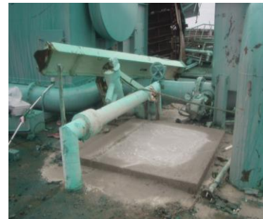
Photograph 3 Blocking of Pits etc.
