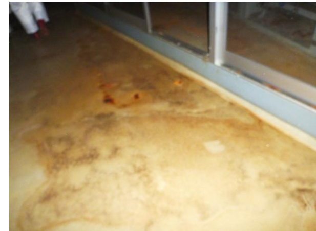
Floor in front of reactor instrumentation rack
