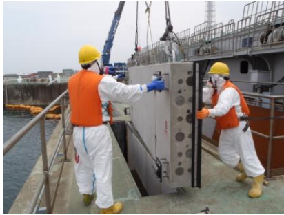
Photograph 1 Installation of Stop-Log
