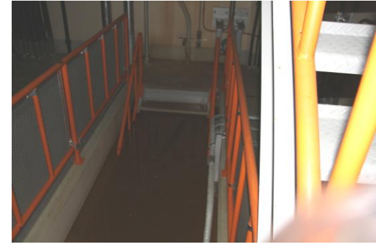
Northwest stairs (half basement)
